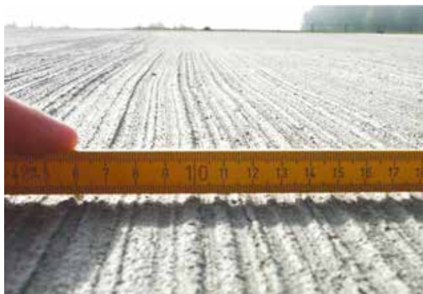
Fig. 6. Concrete surface textured with steel brush
