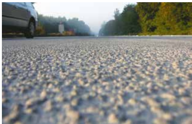
Fig. 5. Concrete surface with exposed aggregate (“waschbeton”)
