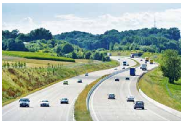
Fig. 2. New section of the A8 Ulm – Augsburg autobahn with cement concrete pavement built under the PPP project
