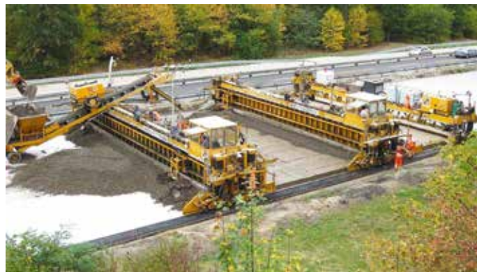
Fig. 8. Concrete laying complex for two-layer concrete placing
